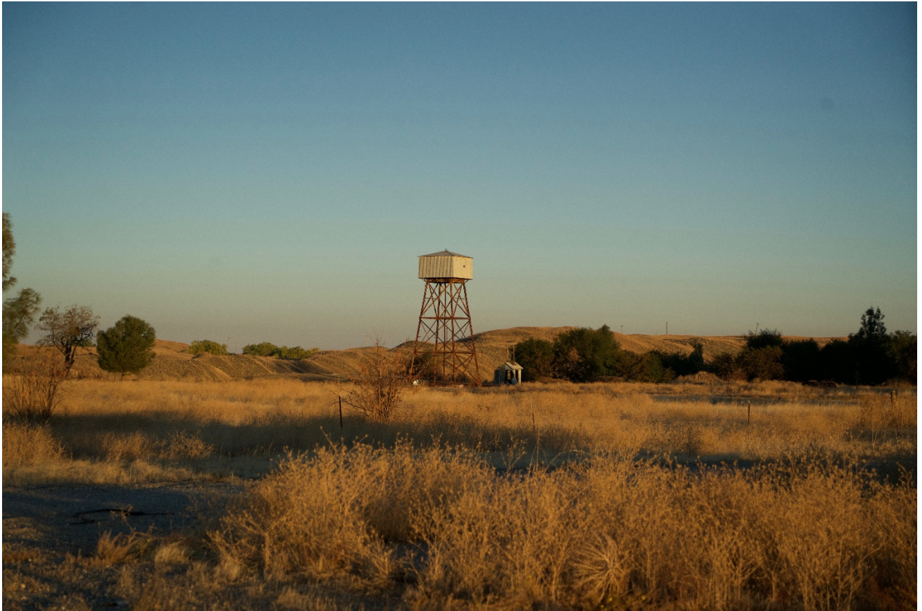
Photo 04: Water tower in the town of Hammonton, CA
