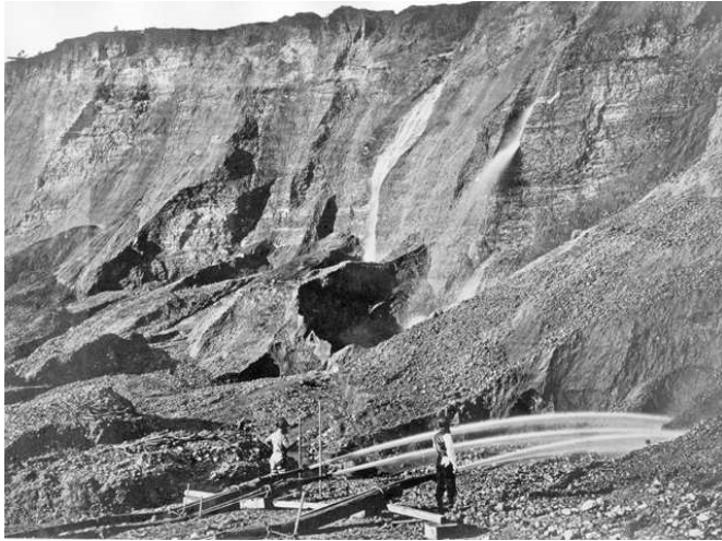
Figure 7 Hydraulic Mining Water Cannon
